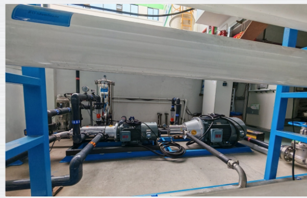
500t/d Seawater Desalination(DHP22 60Bar + HEX(S) -40/60-3)
