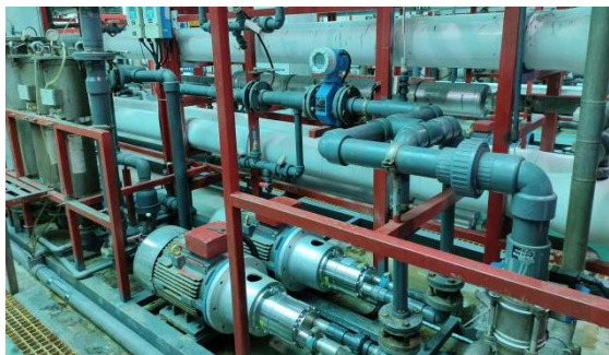
垃圾渗滤液 (DHP8.2, 60bar)
