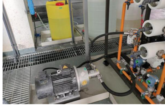
磷酸/硝酸回收 (DHP2.7, 60bar)
